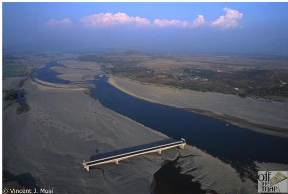
In Honduras, after Hurricane Mitch, the river moved and the bridge was left standing but no longer connected to the river where its' purpose was to be fulfilled.
